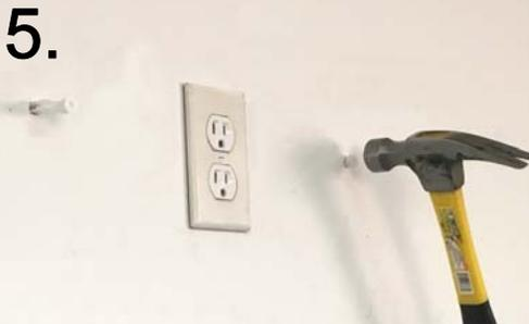
Insert the four plastic keepers that came in the hardware bag into the holes. Using a hammer, lightly tap on the keepers until they are flush with the wall.
