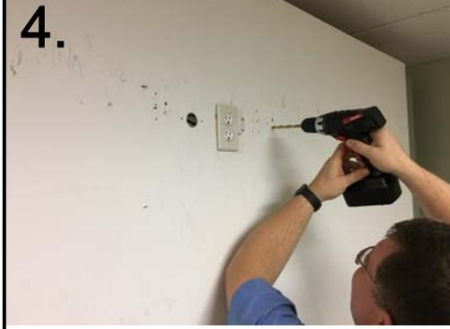
Using the 5/16" drill bit and drill, drill a hole at the four marks on the wall.
