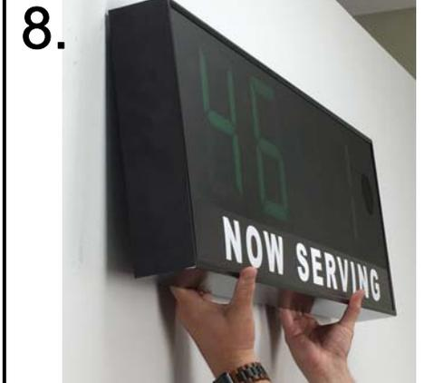
Lift the LED display up above the mounting brackets then ease the display down onto the brackets. Tuck the unused power cord behind the clock and you're finished with install
